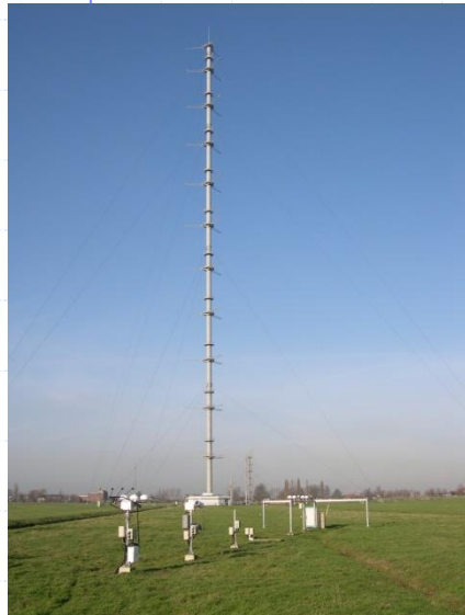
Cabauw tower (KNMI, NL)
